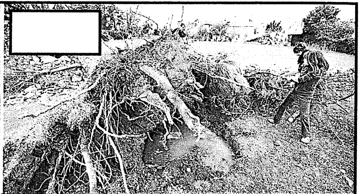
This tornado uprooted a few shallow-rooted trees and damaged many chimneys in the neighborhood.
