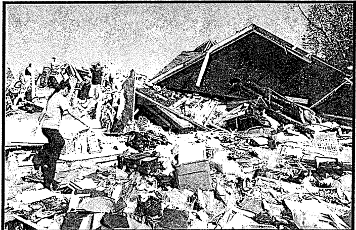
In 2011, a tornado destroyed this house in North Carolina. A tornado warning was issued about 24 minutes before the tornado struck the area.
