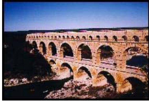
The Roman Aqueduct at Nimes, France. Built in the 1 st Century A.D.
